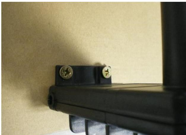
Figure 5: Example of wall mounting
