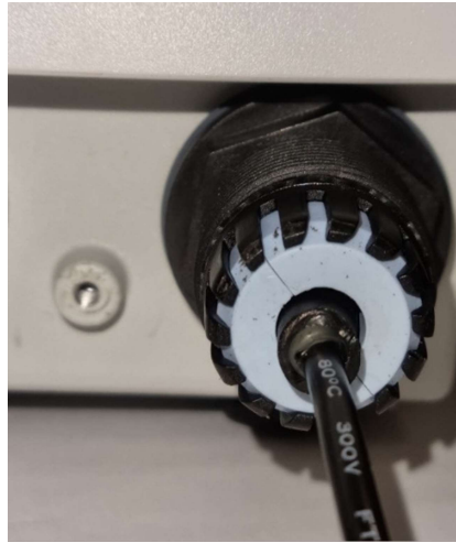
Figure 8: View of the rubber placement
