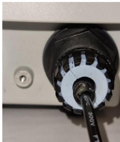
Figure 8: View of the rubber placement
