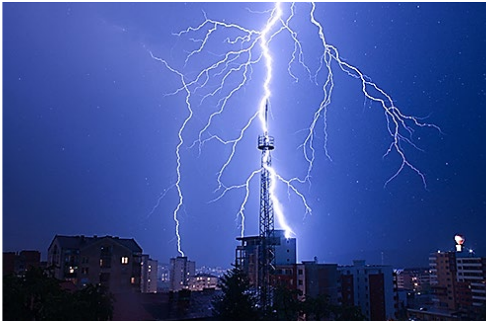
Figure 1 : Lightning strike on a telecommunication tower – Source: CITEI
