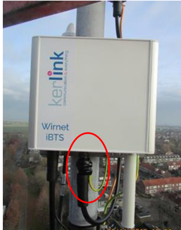
Figure 50 : Example of insulating tape protection on Wirnet iBTS gateway RF port with coaxial lightning protection
