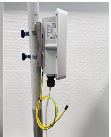
Installation the Wirnet™ iStation on the support
