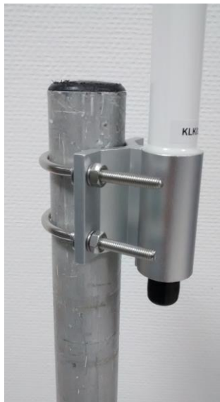
Mount the antenna and U-bolts on the pole
