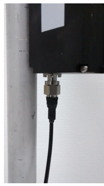
Screw the coaxial cable onto the N connector of the cavity filter
